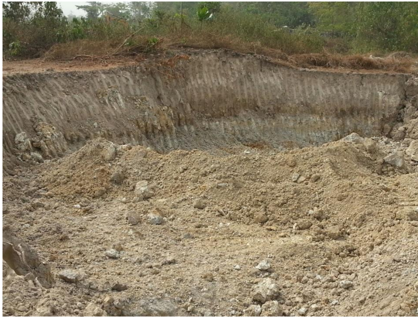
Figure 2: Excavated Pit being backfilled
