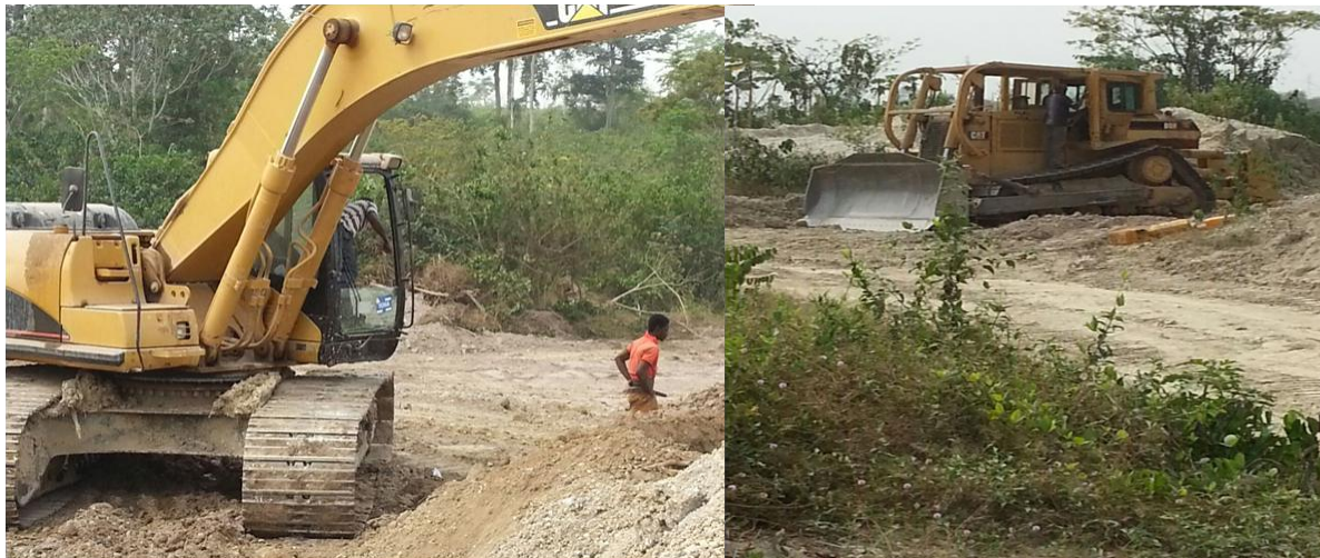
Figure 3: Backfilling using Excavator and Dozer at the Reclamation Site
