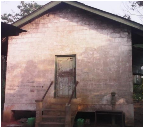
Fig. 2 53-Year Old Compressed Block Structure (Structure has no cracks)
